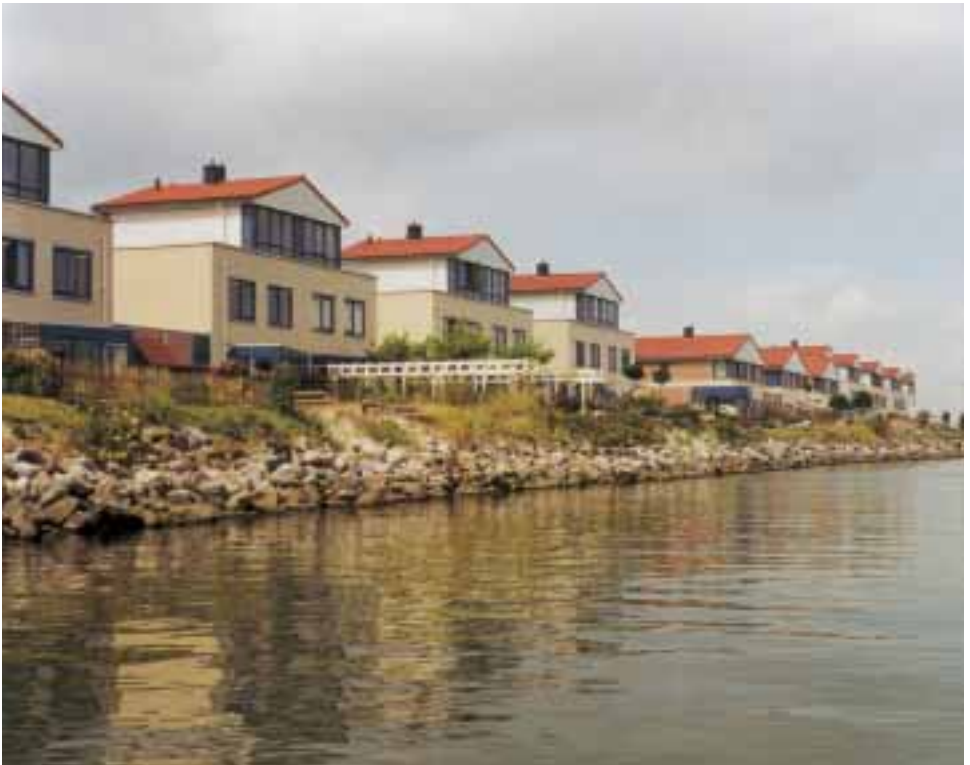
Construction of housing units on the outside of the dike along the IJsselmeer (Photo: RWS-Directorate IJsselmeer area)
