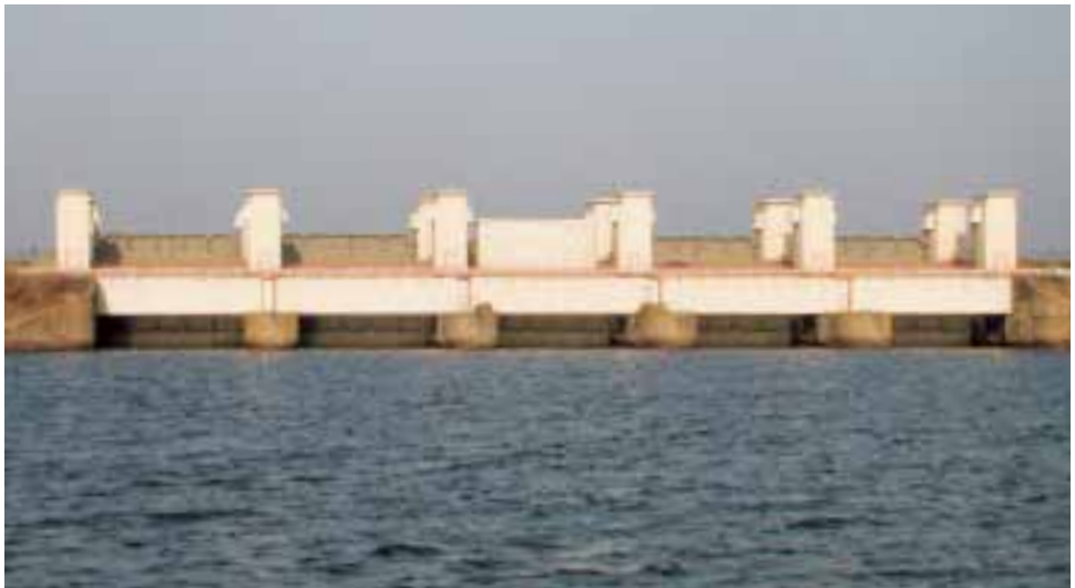
The locks in the Afsluit dike sluice by gravity (Photo: RWS-Directorate IJsselmeer area)
