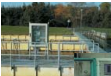
Procescontrole (pH, T, Chloride, geleidendheid e.d.)
