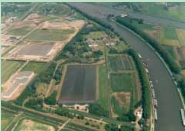
Water supply station along the Lekkanaal near Utrecht.
